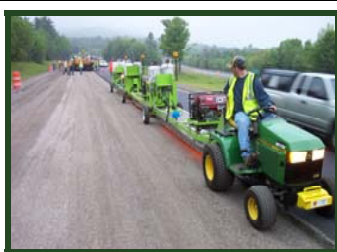
Pre-heaters travel between passing traffic and the paving train.
