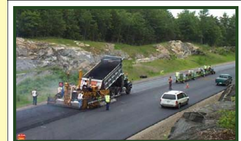
Infrared pre-heater and paver-mounted heater
