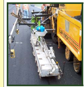
Heater is mounted between the paver and the grade ski.
