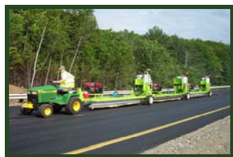
Pre-heaters travel 10-100 feet ahead of the paver
