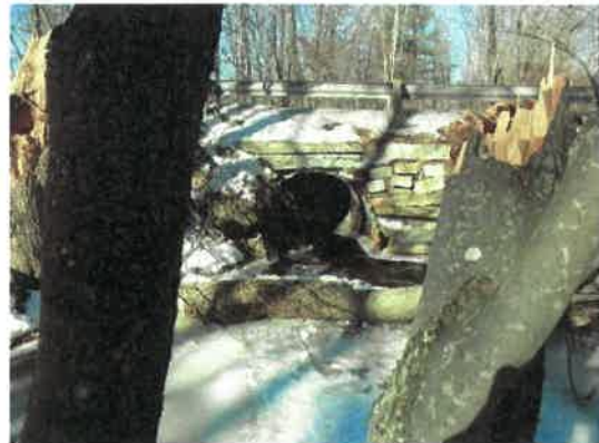
View looking at downstream invert
