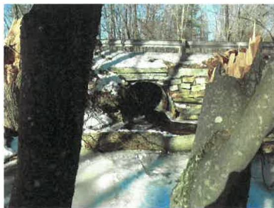
View looking at downstream invert
