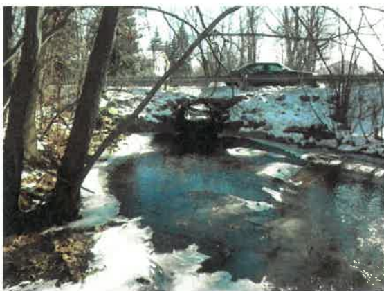
View looking at upstream invert
