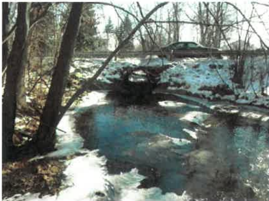
View looking at upstream invert
