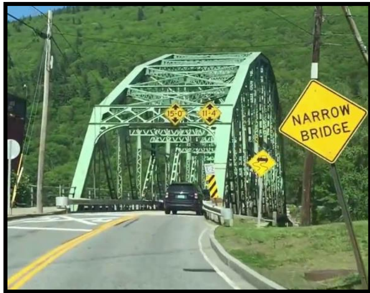
Limited Vertical Clearance and Roadway Width Limit Truck Traffic to One at a Time Crossing the Bridge
