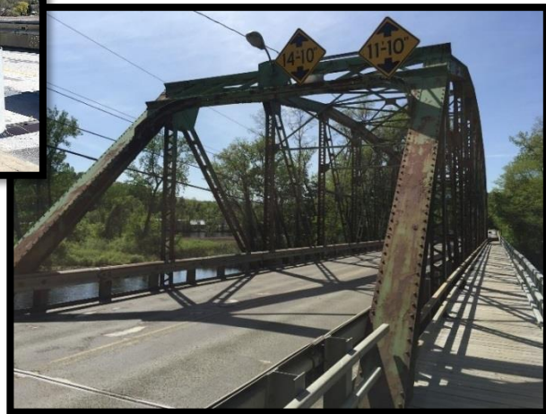
Charles Dana Bridge
