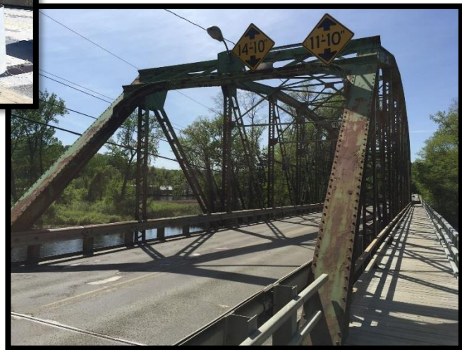
Charles Dana Bridge
