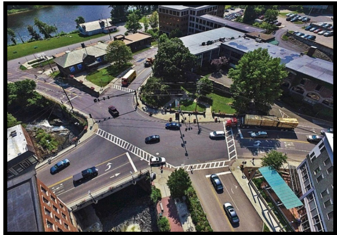
"Malfunction Junction" will be improved by the relocation of Bridge Street to the new alignment of VT Route 119.
