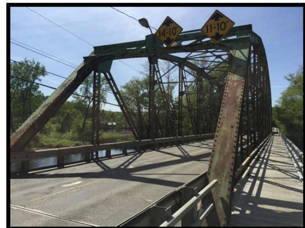
Charles Dana Bridge
