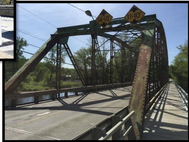
Charles Dana Bridge
