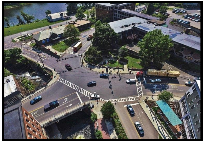
"Malfunction Junction" will be improved by the relocation of Bridge Street to the new alignment of NH Route 119.
