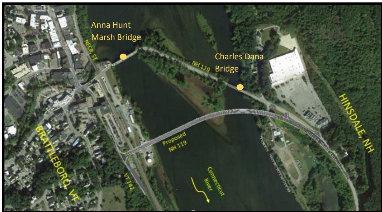
Aerial View of the Existing Bridges Carrying NH Route 119 over the Connecticut River with Proposed Project Location (Looking Upstream/North)
