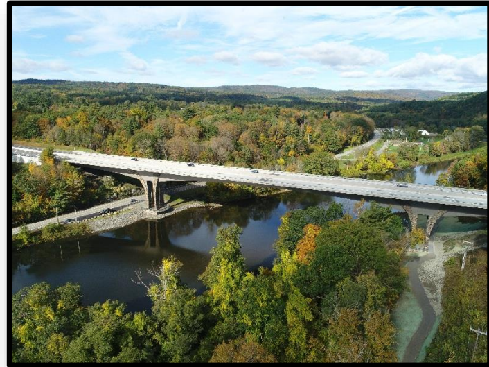
VTrans and FWHA recently invested approximately $60 million to replace the I-91 Bridges over the West River in Brattleboro with the "Bridge to Nature"
