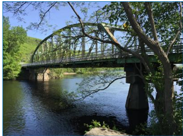
Charles Dana Bridge
