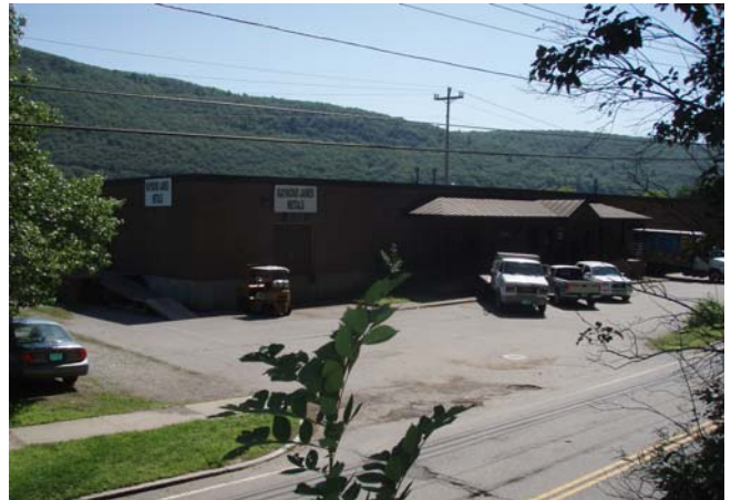
Photo 10 – Blue Seal Building (Front) View of the front of the former Blue Seal building (VT touchdown area) from VT 142 southeast towards New Hampshire.
