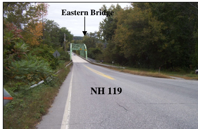
Photo B-2 Eastern Bridge: View from Route 119 in Hinsdale west towards the mid-channel island.
