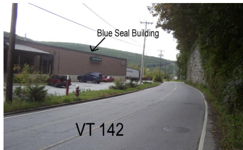
Photo D-1 Blue Seal Building: View from VT 142 looking south.
