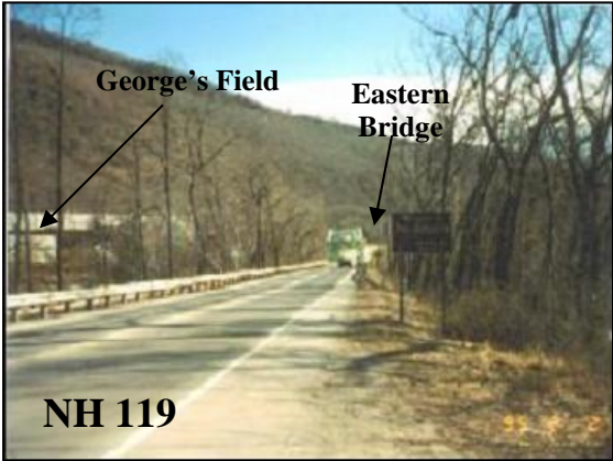
Photo B-5 NH 119: View from the mid-channel island east towards the eastern bridge.
