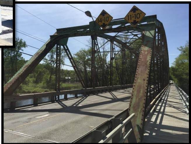
Charles Dana Bridge
