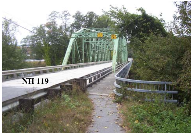
Photo PS -2 Eastern Bridge: View from New Hampshire, west towards the Mid-channel Island and Brattleboro
