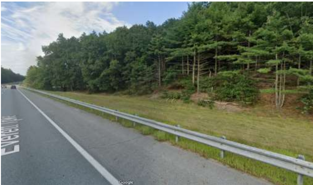
Photo 8: Impact Location I (PS) East Side of FEET South of Pennichuck Brook Crossing
