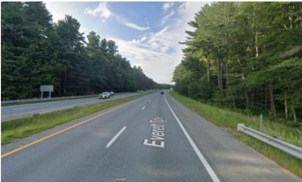
Photo 14: Impact Location M (NWB) North of Pennichuck Brook Crossing
