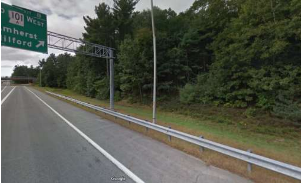
Photo 3: Impact Location C (PS) West Side of FEET
