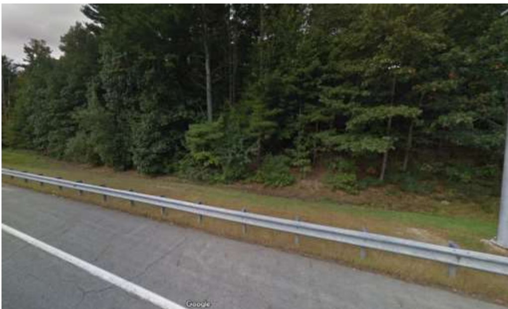
Photo 2: Impact Location B (NWB) West Side of FEET
