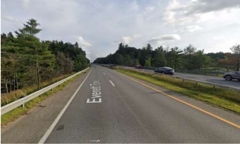
Photo 13: Impact Location L (WB) and M (NWB) North of Pennichuck Brook Crossing
