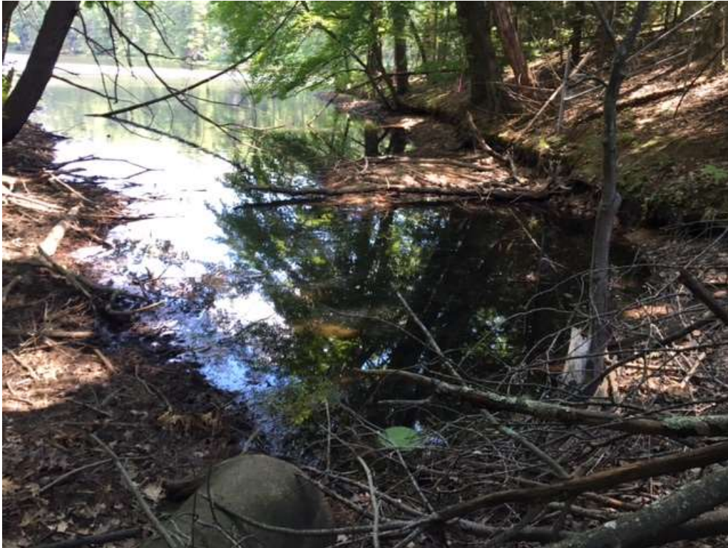
Photo 7: Impact Locations F, G, and H (WB) Drainage Outlet at Harris Pond
