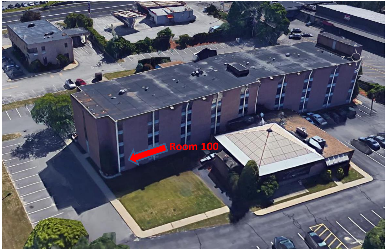
Diag. A (Satellite Image of the Northwest Corner of Quality Inn)
