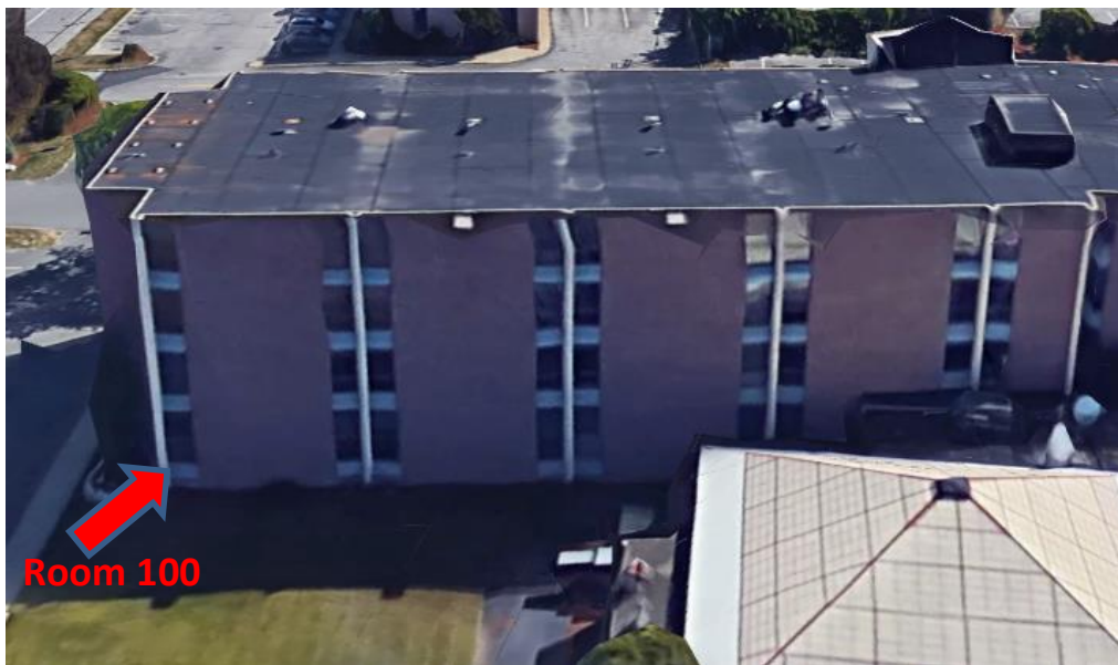
Diag. D (Satellite Image of West Side of Quality Inn)
