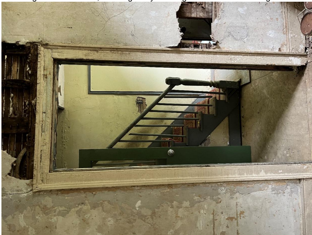
Photo # 15: Interior, Rixford House, showing typical door casing. Main staircase and newel post in background. Looking NW.
