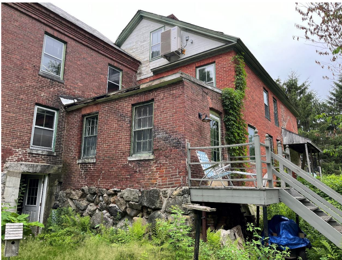
Photo # 8: Conjoining addition, looking E.
