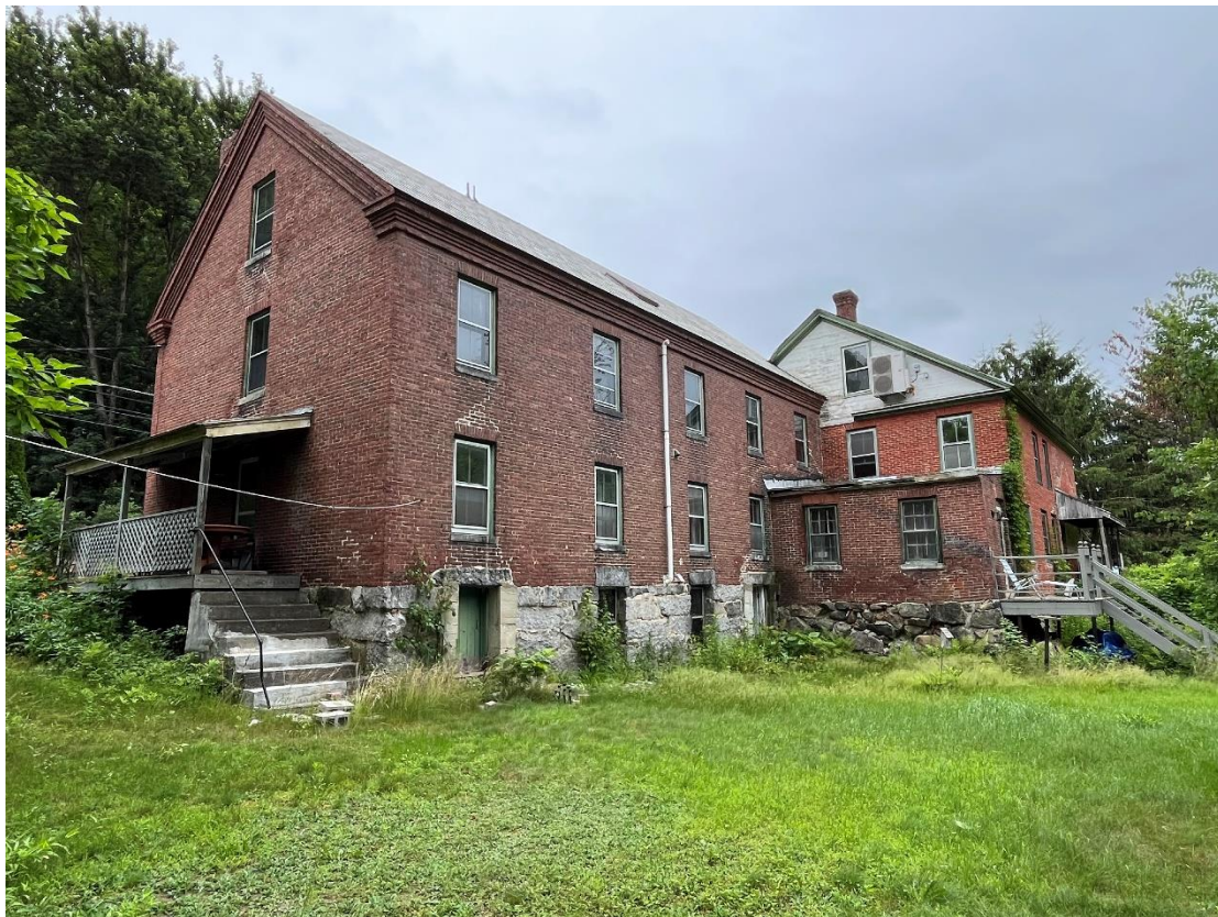
Photo # 7: Rear of boarding house wing, looking E.
