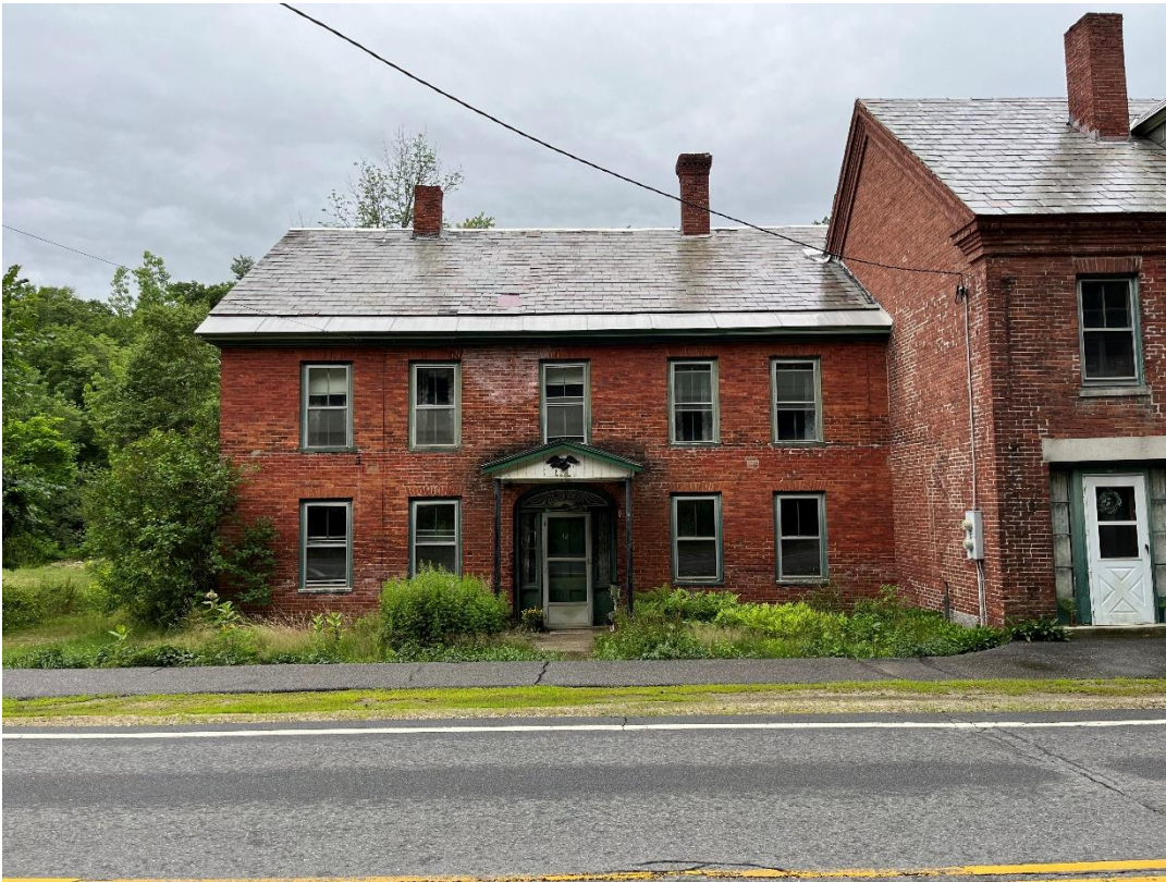
Photo # 2: Façade of Rixford House, looking SW.
