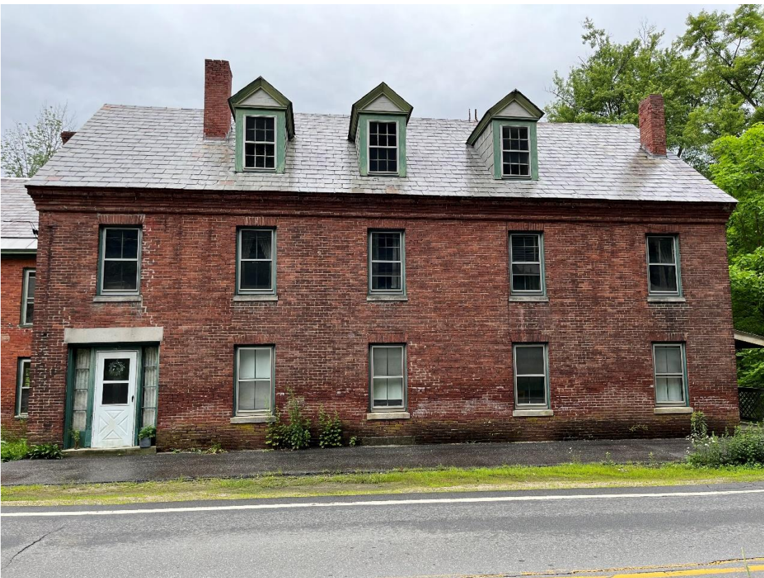
Photo # 3: Façade of boarding house wing, looking SW.
