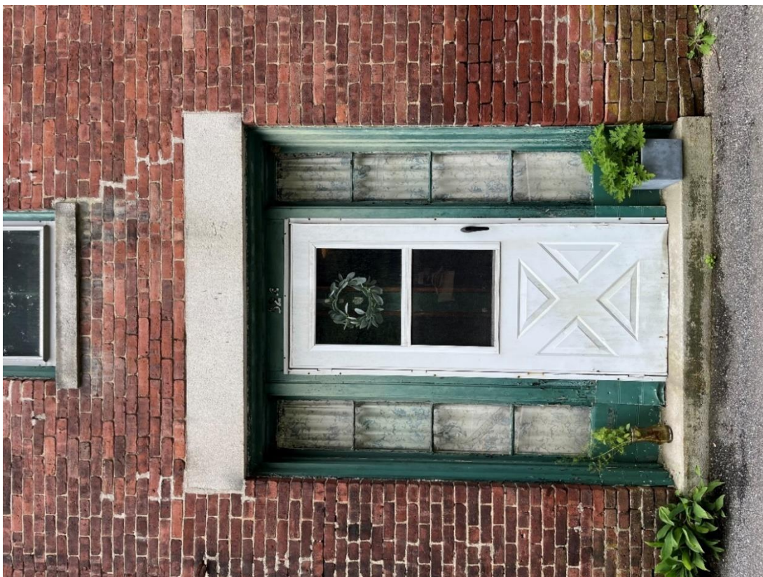
Photo # 14: Boarding house entrance, showing finely tooled granite header. Looking SW.
