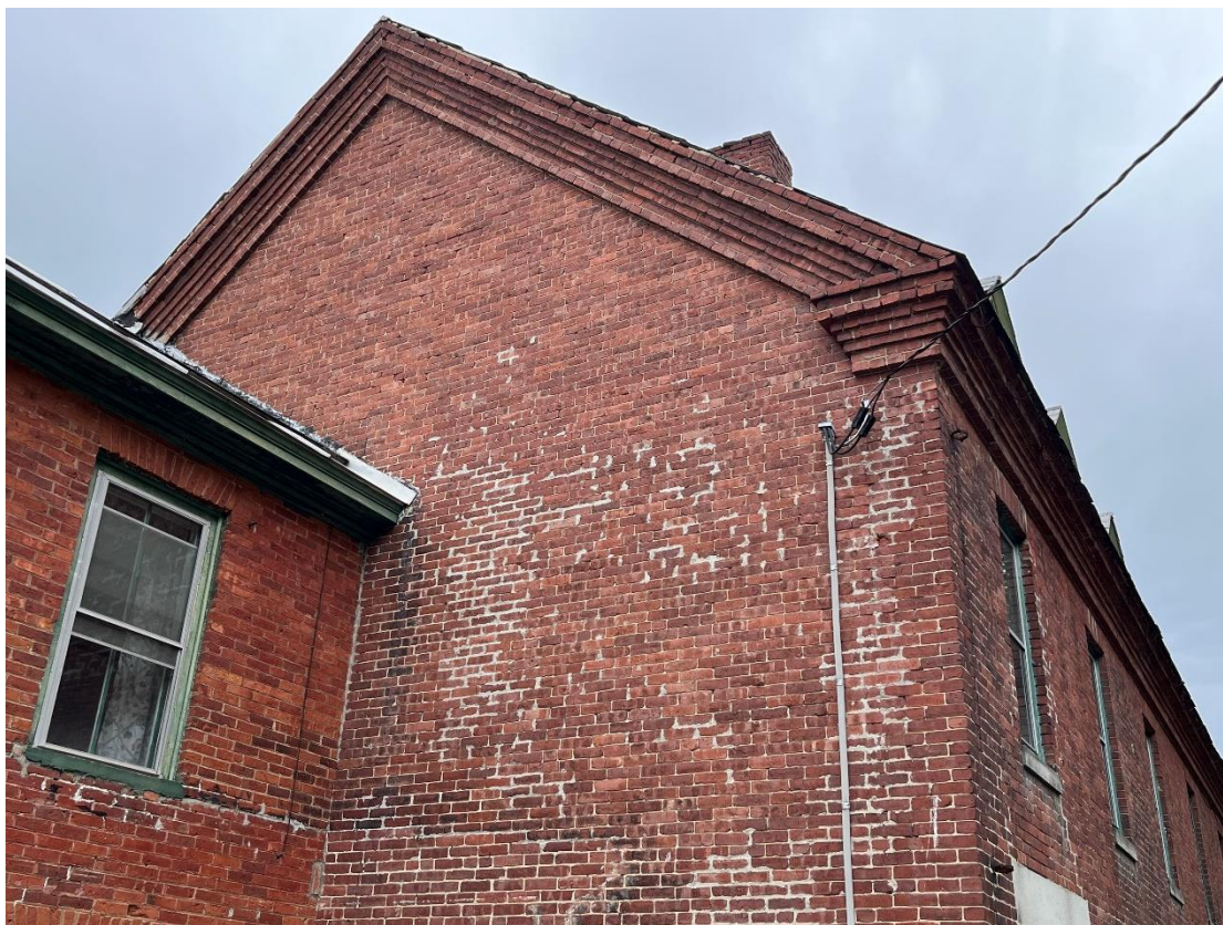
Photo # 11: Detail of periscoping cornice at the boarding house wing. Looking NW.
