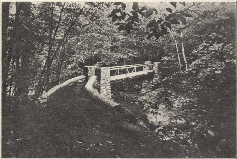
Pathmakers' Memorial Bridge, Randolph, N. H. Facing East on the "Link Path"
