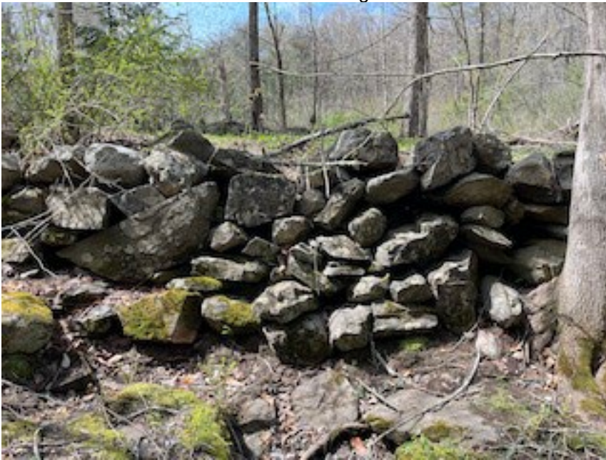
Photo #2 East side of east wall taken facing west. 5/6/24
