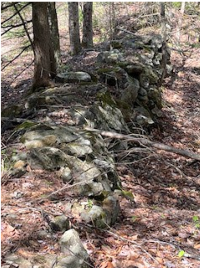
Photo #3 South end of east wall facing north. 5/6/24
