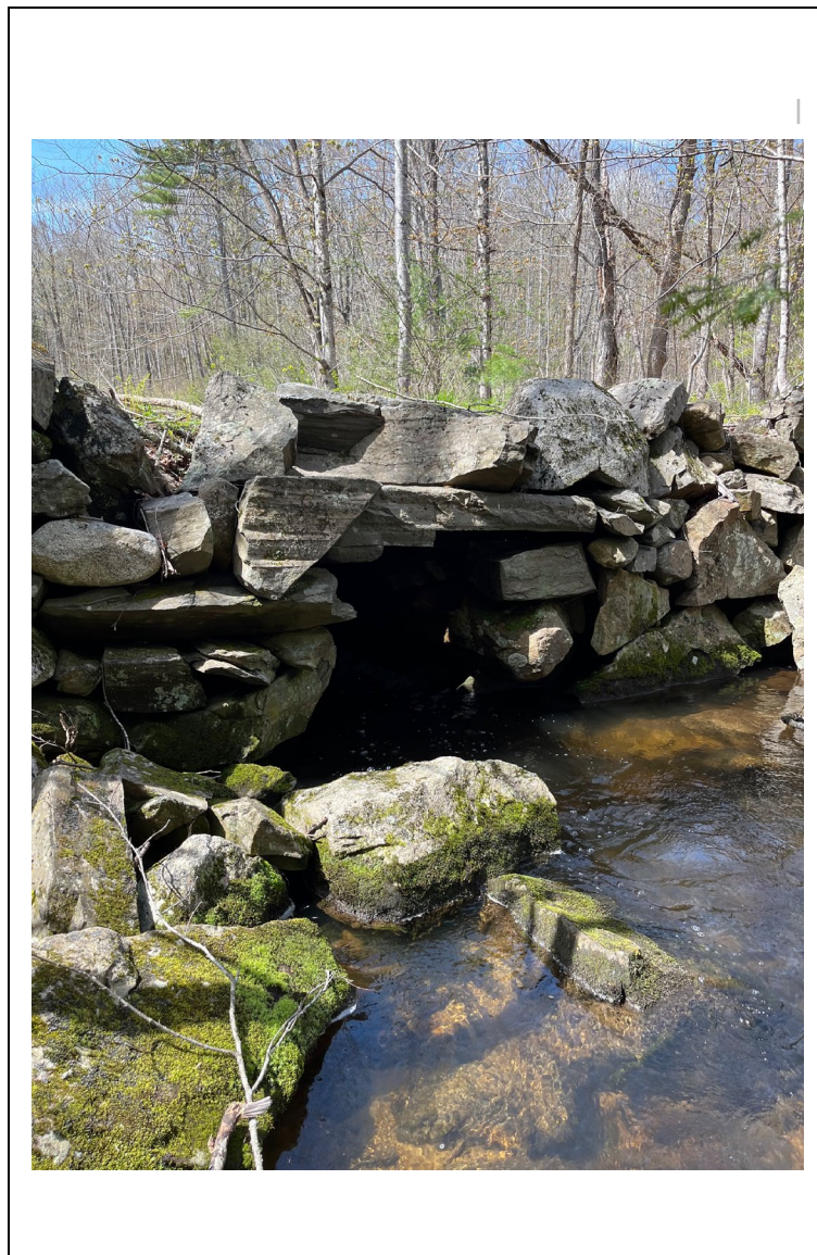
Photo #1 east wall of culvert and causeway. 5/6/24
