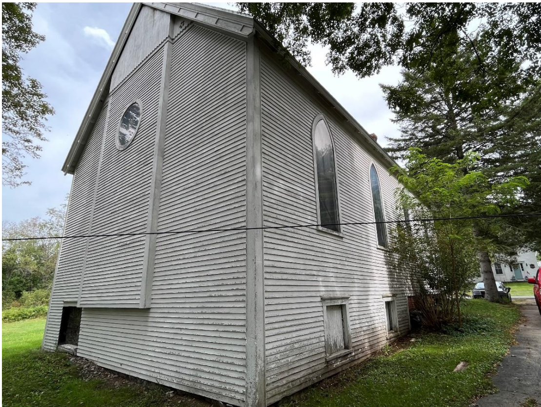
Photo # 3. Looking NE, showing the rear and southern elevation.
