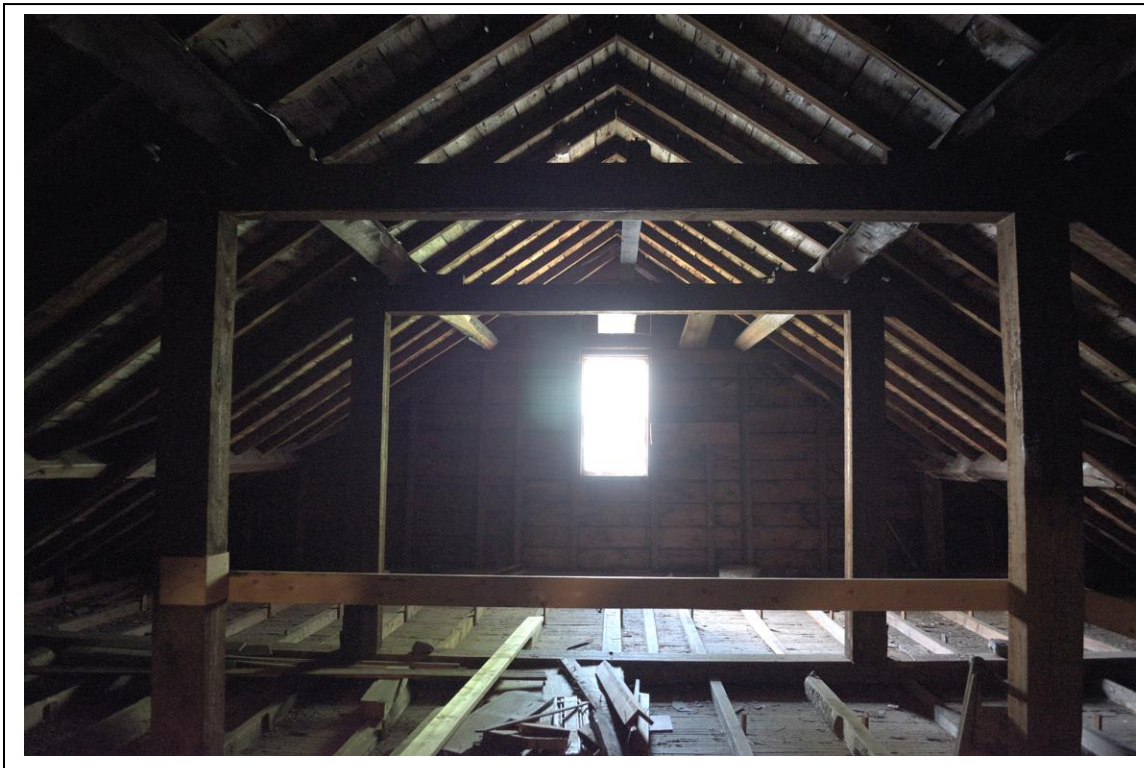
Photo # 9 Description (with direction): Exposed 1844 frame in attic, facing southwest
