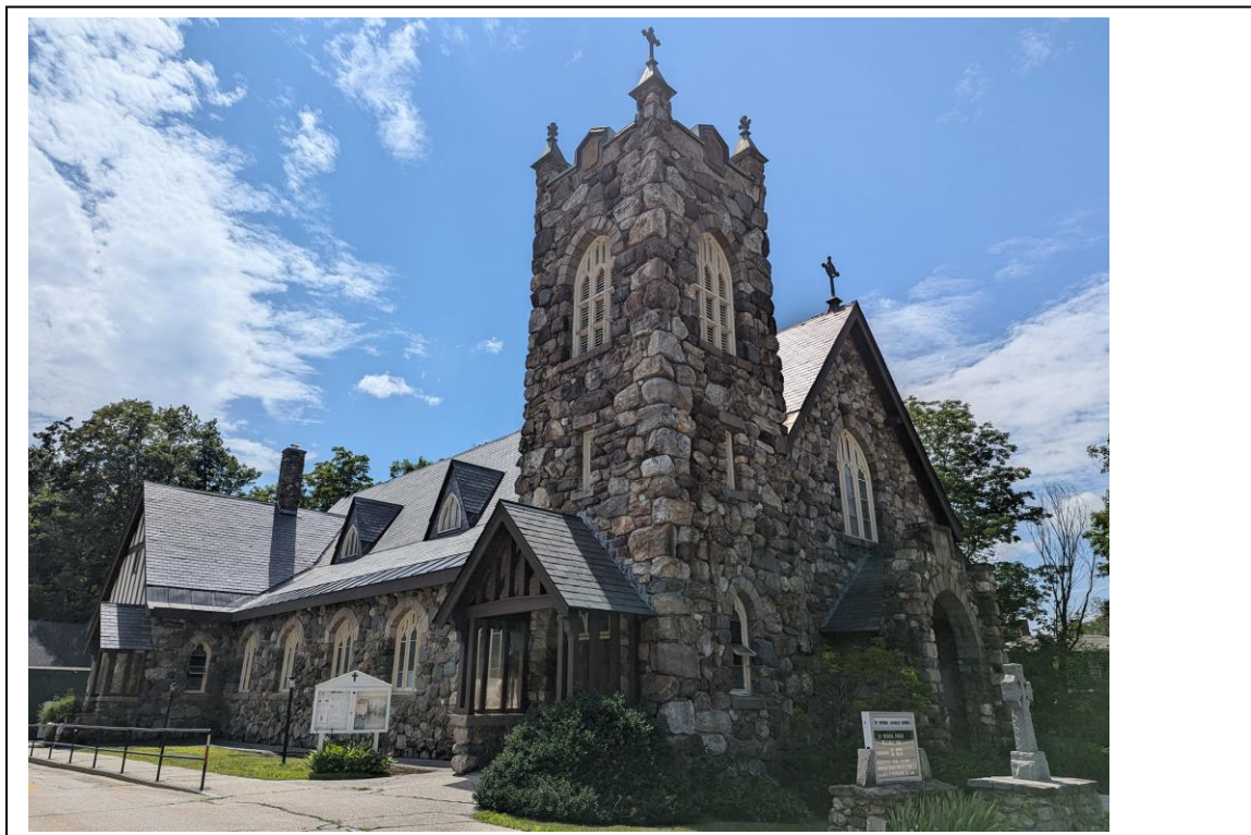
Photo # 13 Description (with direction): The Gothic Revival field-stone St. Patrick's Catholic Church in East Jaffrey was built at what is now 87 Main Street in 1916-1917. Photograph facing southwest.
