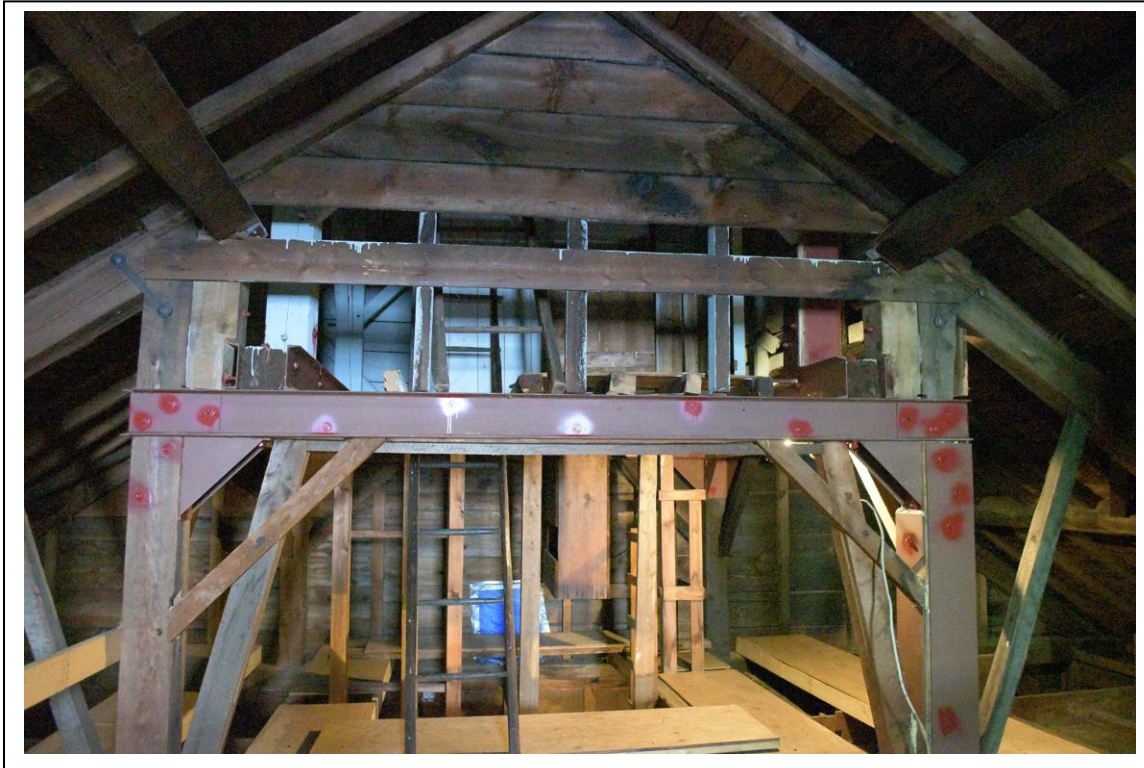
Photo # 10 Description (with direction): Belfry framing with ca. 1994 metal sub-structure, facing northeast
