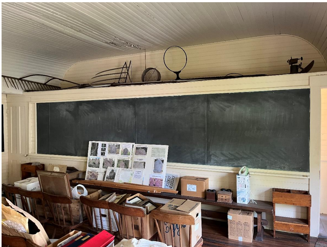
Photo # 10 Description (with direction): Interior, second floor, looking SW toward front and 1908 blackboard.
