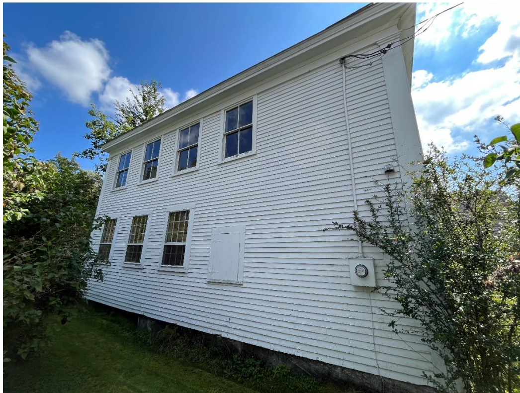
Photo # 6 Description (with direction): North elevation, looking SE.
