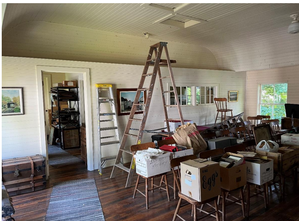
Photo # 9 Description (with direction): Interior, second floor, looking east toward c.1990 partition.
