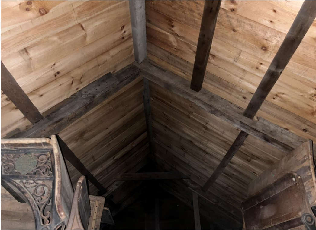
Photo # 8 Description (with direction): Attic, showing roof framing. Looking SSW
