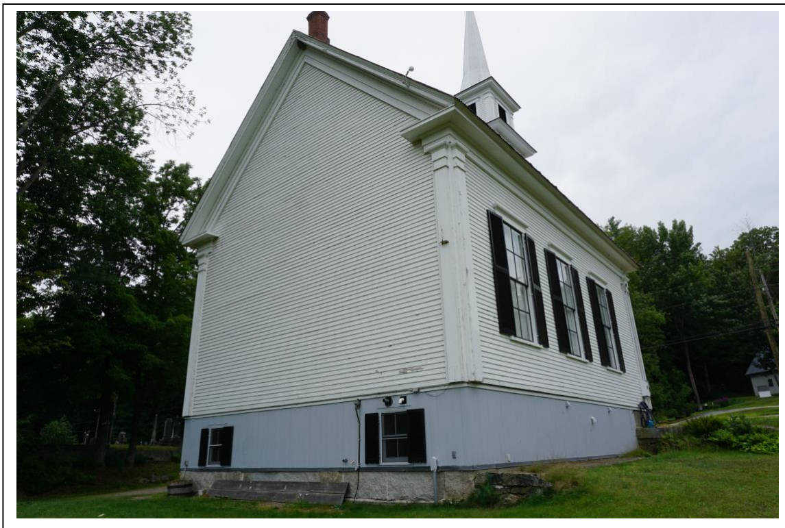
Photo #3 Description: View looking south at rear and west elevations
